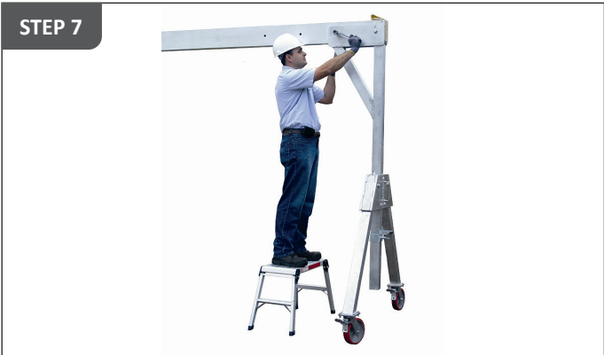
Insert the pins and tighten everything
